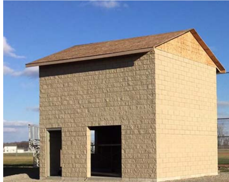
Progress to date (actual site picture)
